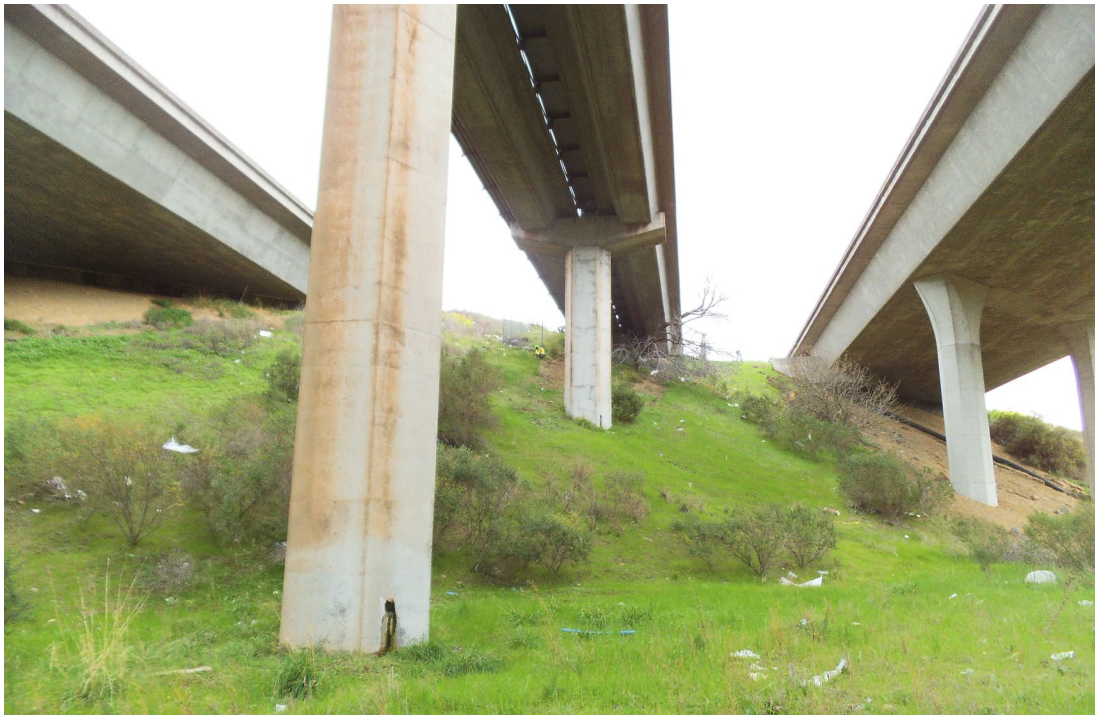
Note: Project site is the middle structure and the slope below, as viewed from Kinne Blvd., looking west. Figure 10. View of Concord Project Site C3015W
