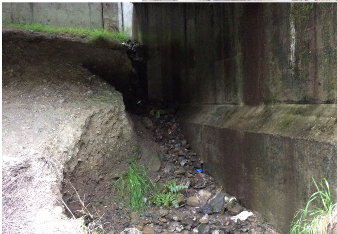
Figure 8. Views of Erosion and Drainage Problems at Castro Valley Project Sites
