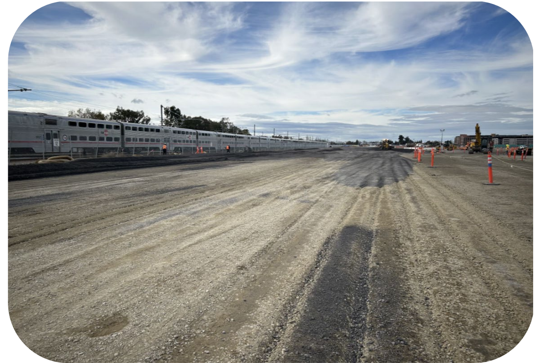
Grading complete for top of launch structure.
