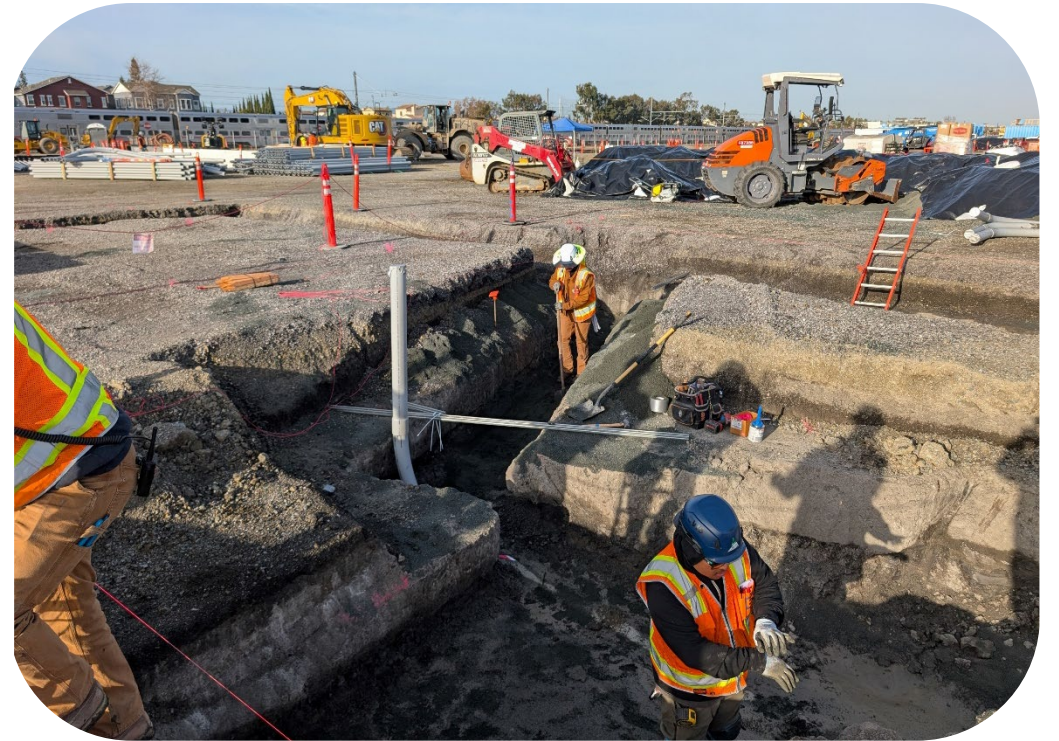
Installing lateral utility connections.
