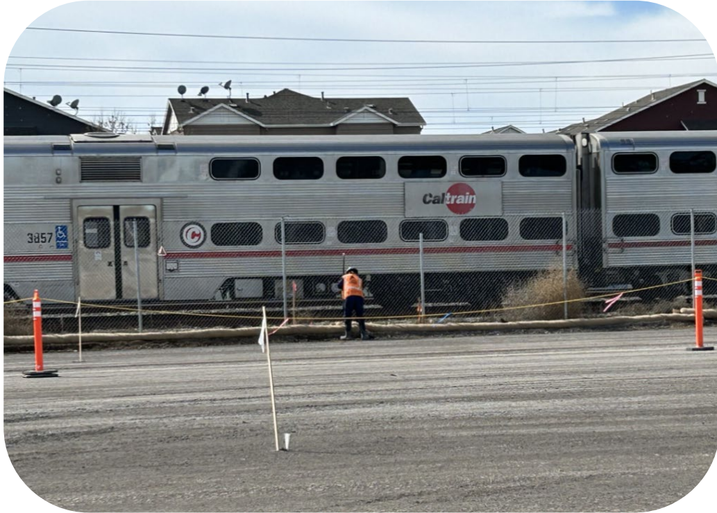
Survey checks for instrumentation and monitoring.
