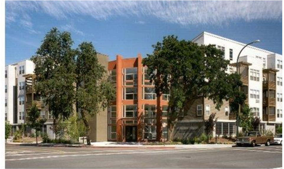
Coggins Square Affordable Apts., Pleasant Hill BART Photo credit: BRIDGE Housing
