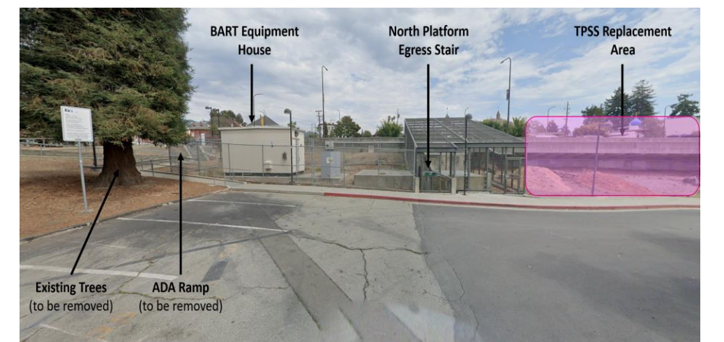
From Parking Lot
