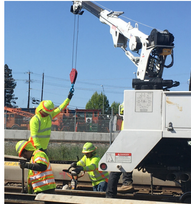
BART often utilizes cranes and forklifts to move oversized track components during weekend shutdowns.
