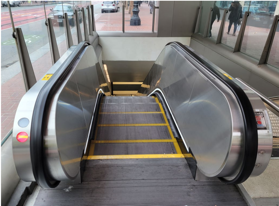
Completed Escalator at Powell St. Station
