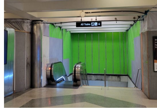
Coordination with BART Projects Substation Project Coordination at Montgomery St. Station
