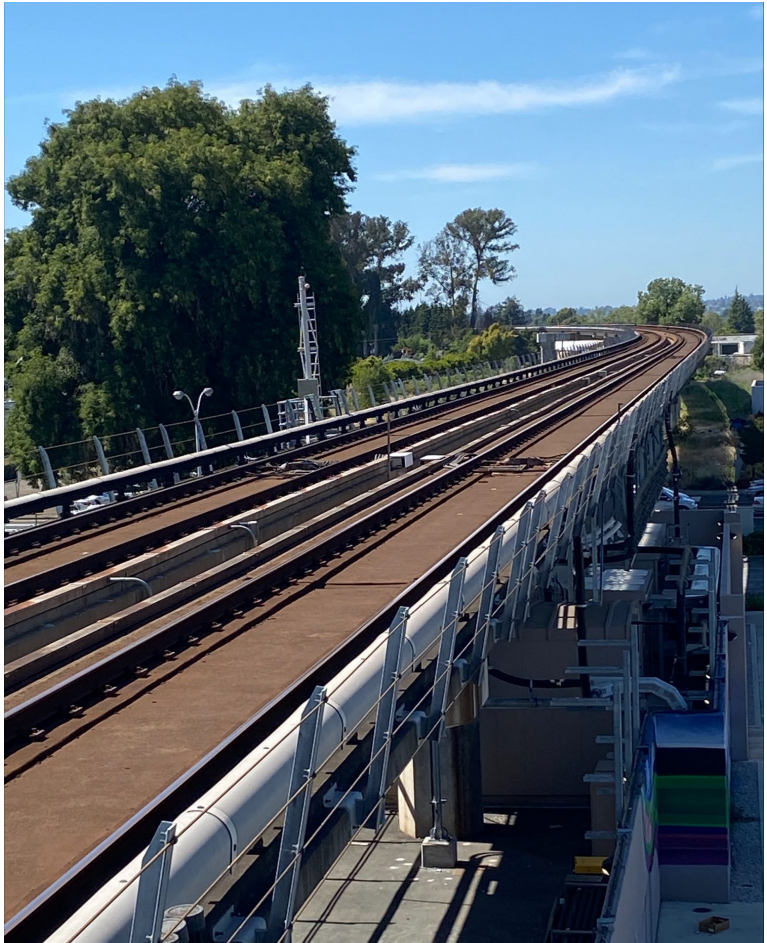
Completed A-Line Aerial Fall Protection at San Leandro BART Station (A40)
