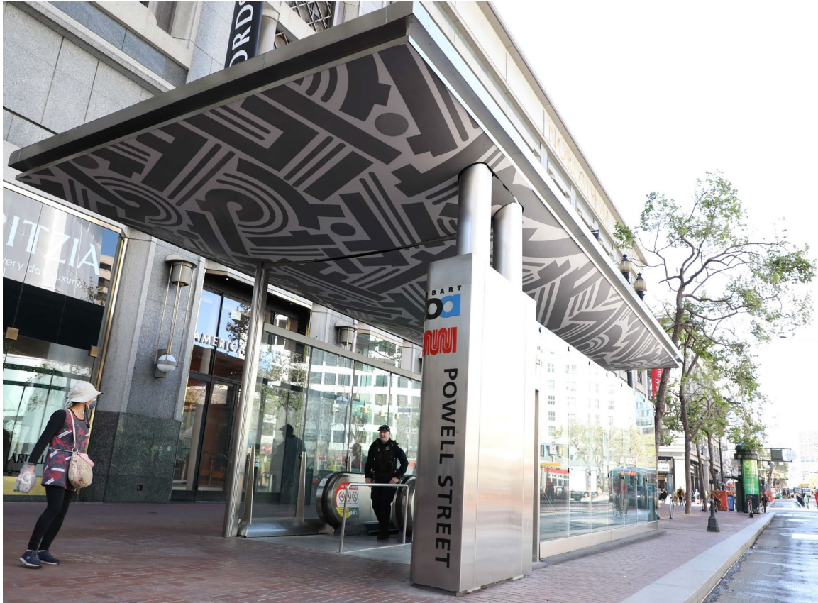
Completed Canopy at Powell St. Station
