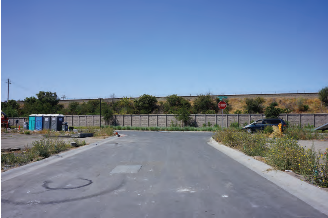
Photo 5: View 3 - Existing Conditions
