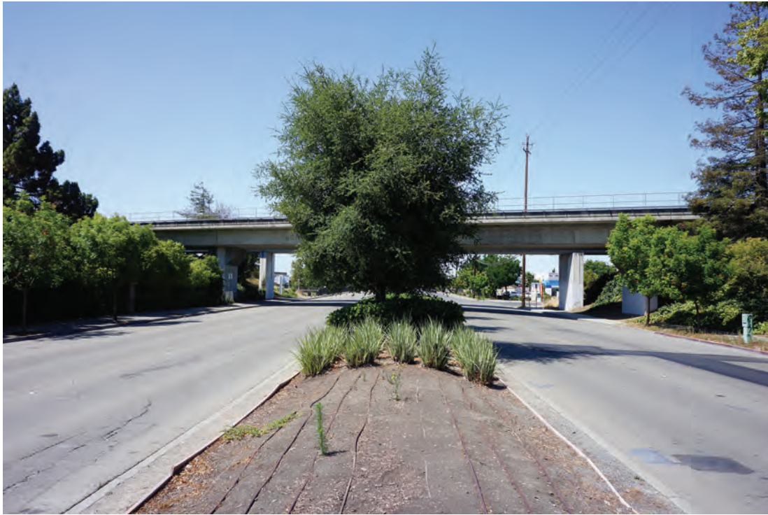
Photo 1: View 1 - Existing Conditions
