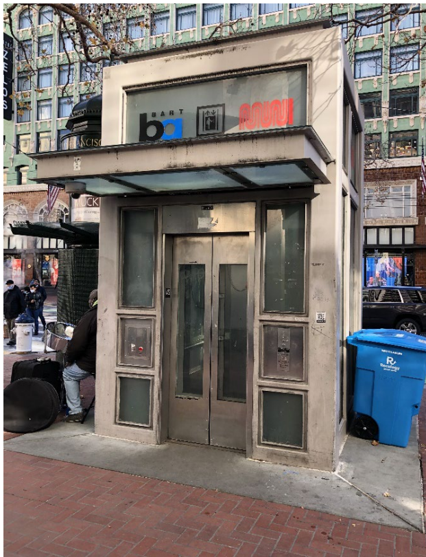
Figure 5. Street elevator at Powell St. Station, December 2021.
