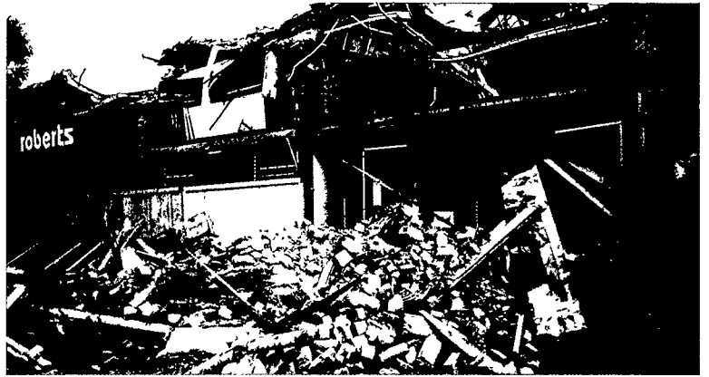
15-8 Example of damage in the historic Pacific Garden Mall area in Santa Cruz, a tourist destination with many small businesses, Loma Prieta earthquake, 1989.
