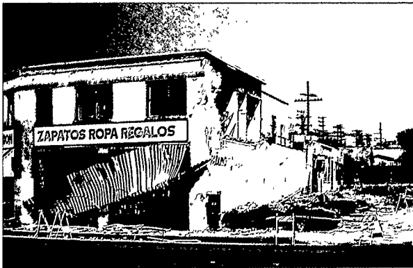
10-10 Damage to unreinforced masonry and wood-frame storefront buildings, Whittier Narrows earthquake, 1987.
