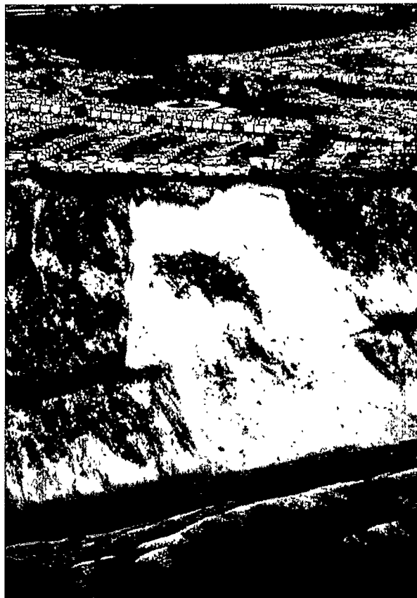
3-14 Landslide failure along the coastal bluffs in the Daly City area.
