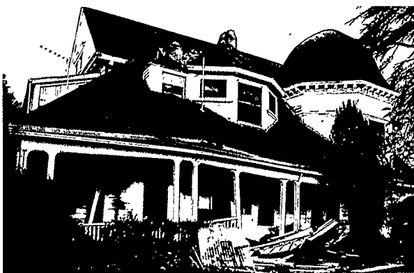
10-11 An old wood-frame house that shifted off its foundation as a result of the failure of cripple stud walls, Loma Prieta earthquake, 1989.
