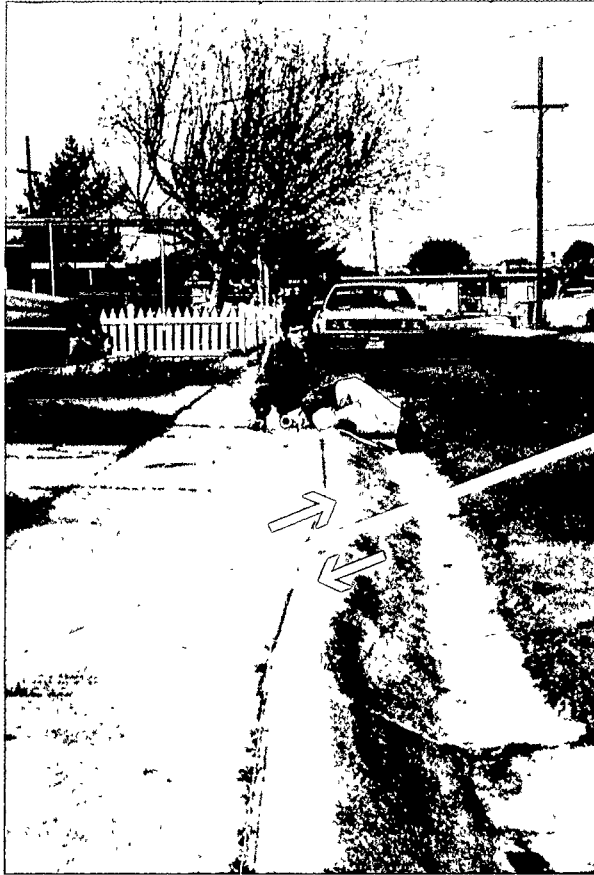
2-8 Sidewalk offset by creep along the Hayward fault in San Pablo.
