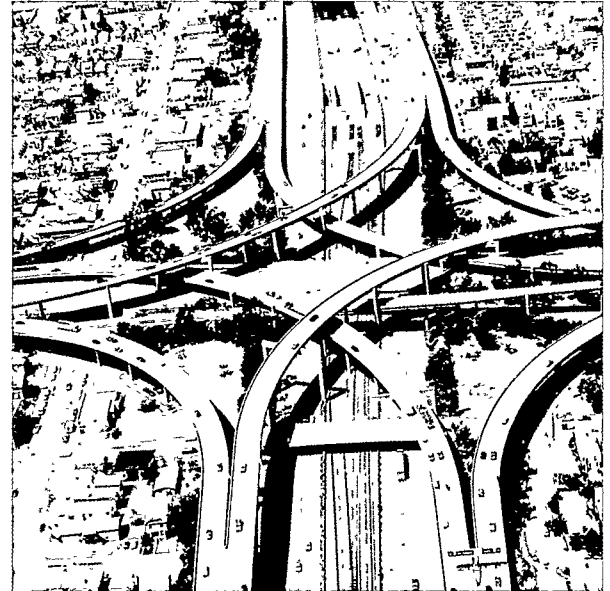
7-10 Aerial view of the Interstate 580-980-24 interchange.
