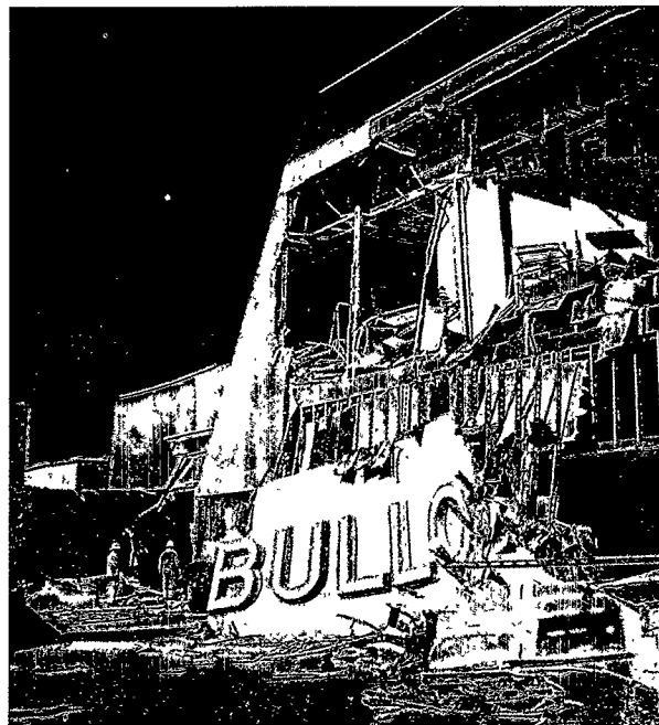
10-2 Damage to Bullock's department store in the Northridge Fashion Center, Northridge earthquake, 1994. LA TIMES PHOTO
