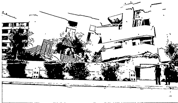
10-3 Damage to wood-frame, multifamily residential buildings, Northridge earthquake.
