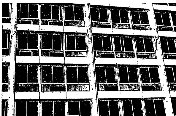
10-13 Shear failure of columns in a nonductile concrete-frame hotel structure in Van Nuys, Northridge earthquake.
