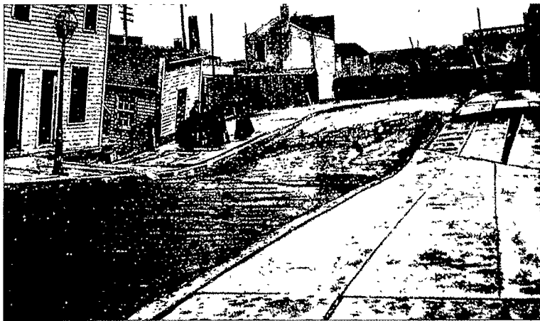
3-11 Settlement from liquefaction and compaction of material in San Francisco following the 1906 earthquake.
