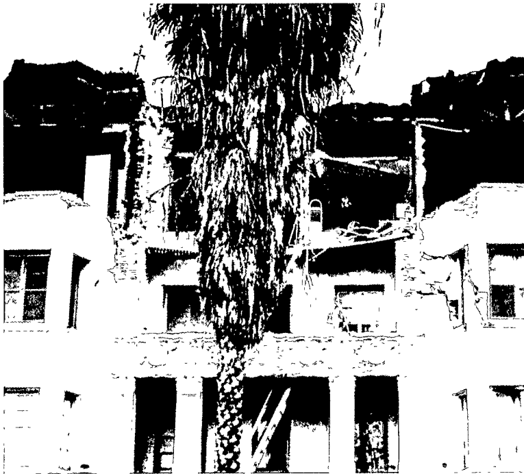
11-3 Apartment house in Santa Monica damaged in the Northridge earthquake, 1994.
