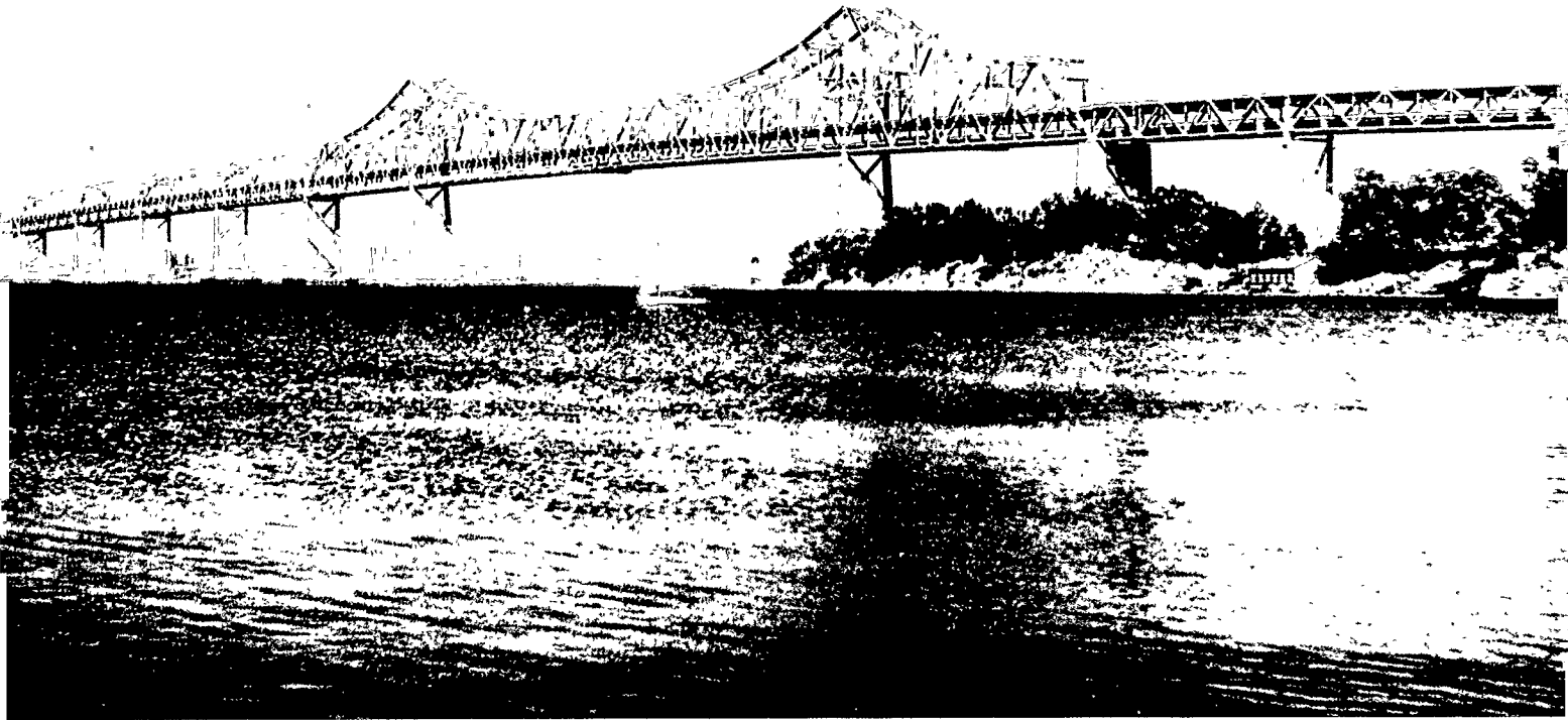
7-1 The San Francisco–Oakland Bay Bridge: east span (top) from Yerba Buena Island to Oakland, truss and cantilever sections; west span (bottom) from San Francisco to Yerba Buena Island, suspension section.
