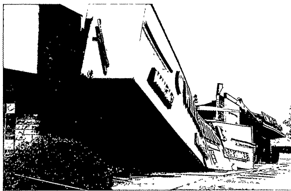
10-4 Damage to downtown strip shopping mall, Northridge earthquake.
