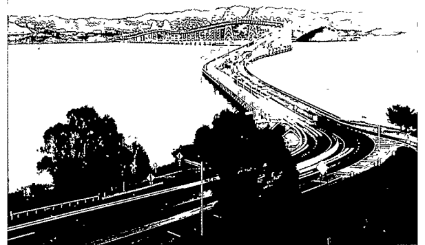
7-5 The Richmond–San Rafael Bridge.
