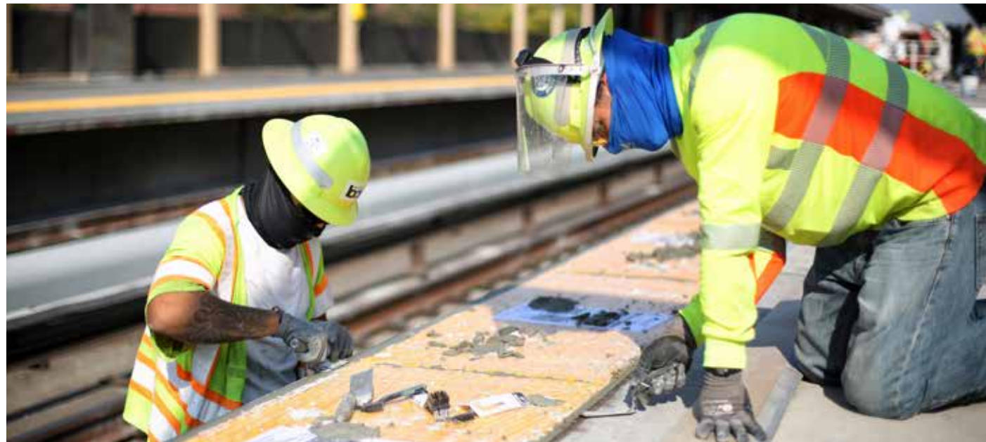
Platform edge tile replacement work at Hayward Station.
