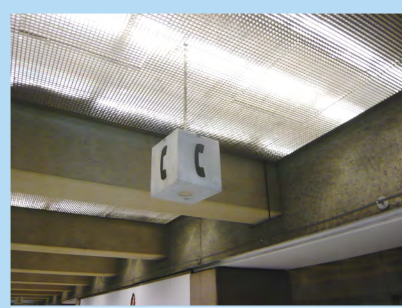
Modernize outdated light fixtures
