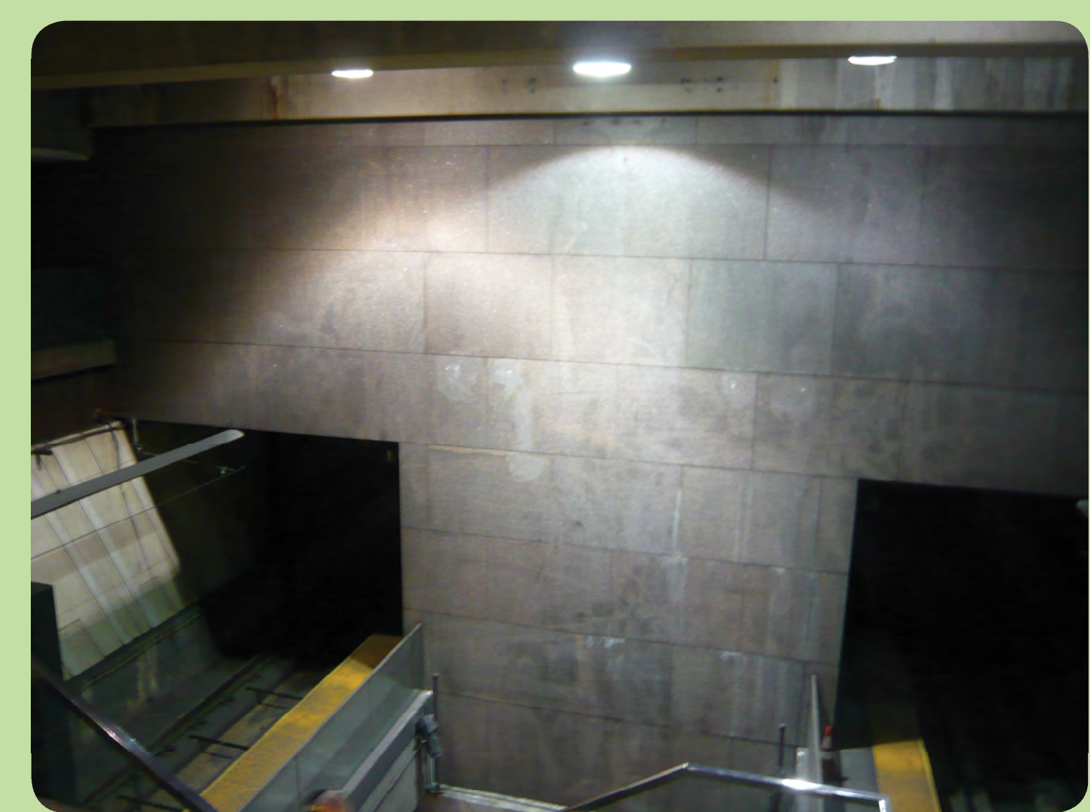
A potential location for the new elevator.
